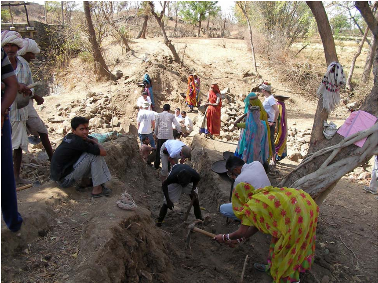
Figure 3 Digging a trench for a subsurface river dam
