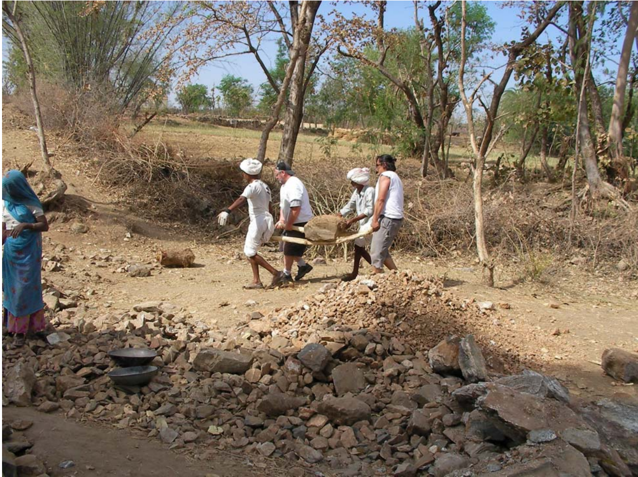
Figure 7 Joining in to move rocks into the dam
